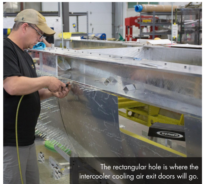
Hunter works on the lower right fuselage skin. This one is the most forward of the large skin sections.
